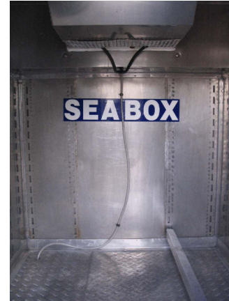
Stainless Steel lining
